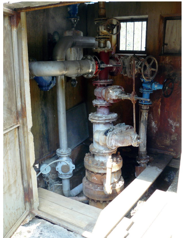
Fig. 1.5 Wellhead of borehole OZ-1 (left) and OZ-2 (right) Oravice (Photo: Marcin, 2013)
